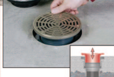
INSTALL FINISH FIXTURE & ADJUST
