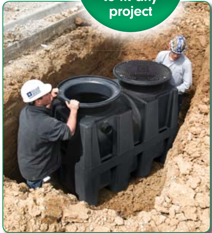
Photo Series: GB-250 installed inside failed precast interceptor (McDonalds)
