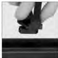
Insert base, twist and lock into strut channel.
