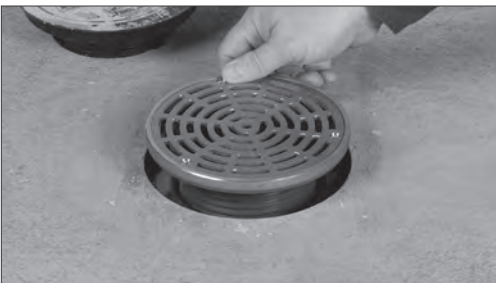
Install Finish Fixture
