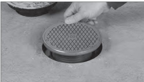
Install Finish Fixture
