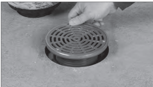
Install Finish Fixture
