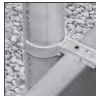
Secure pipe to form for stack placement inside stud wall.
