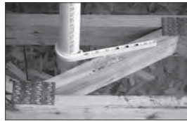
Locking finger allows installation at all angles.
