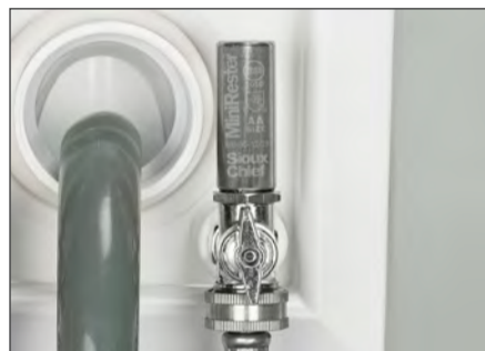
Optional MiniRestor™ provides code-required protection for appliances with quick-closing valves
