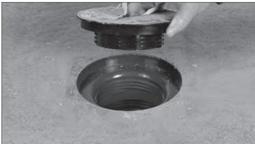
Remove Coring Plug
