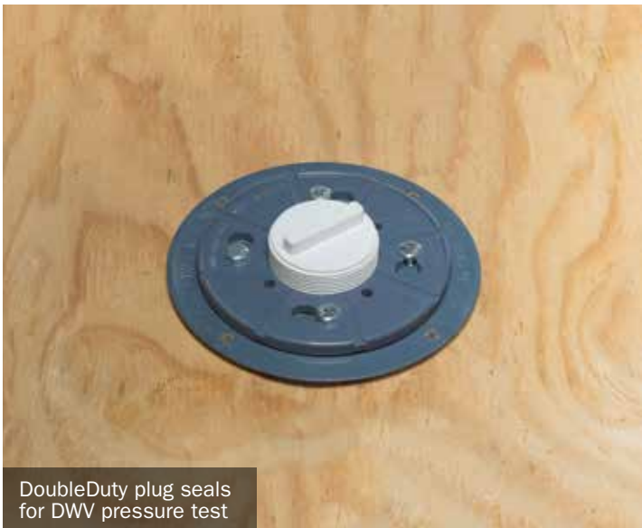
Install round-to-square adapter
