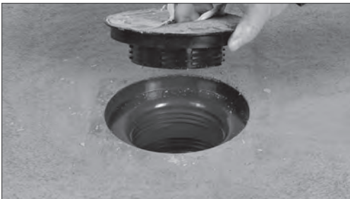
Remove Coring Plug
