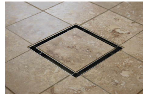
Tile-In drain installation
